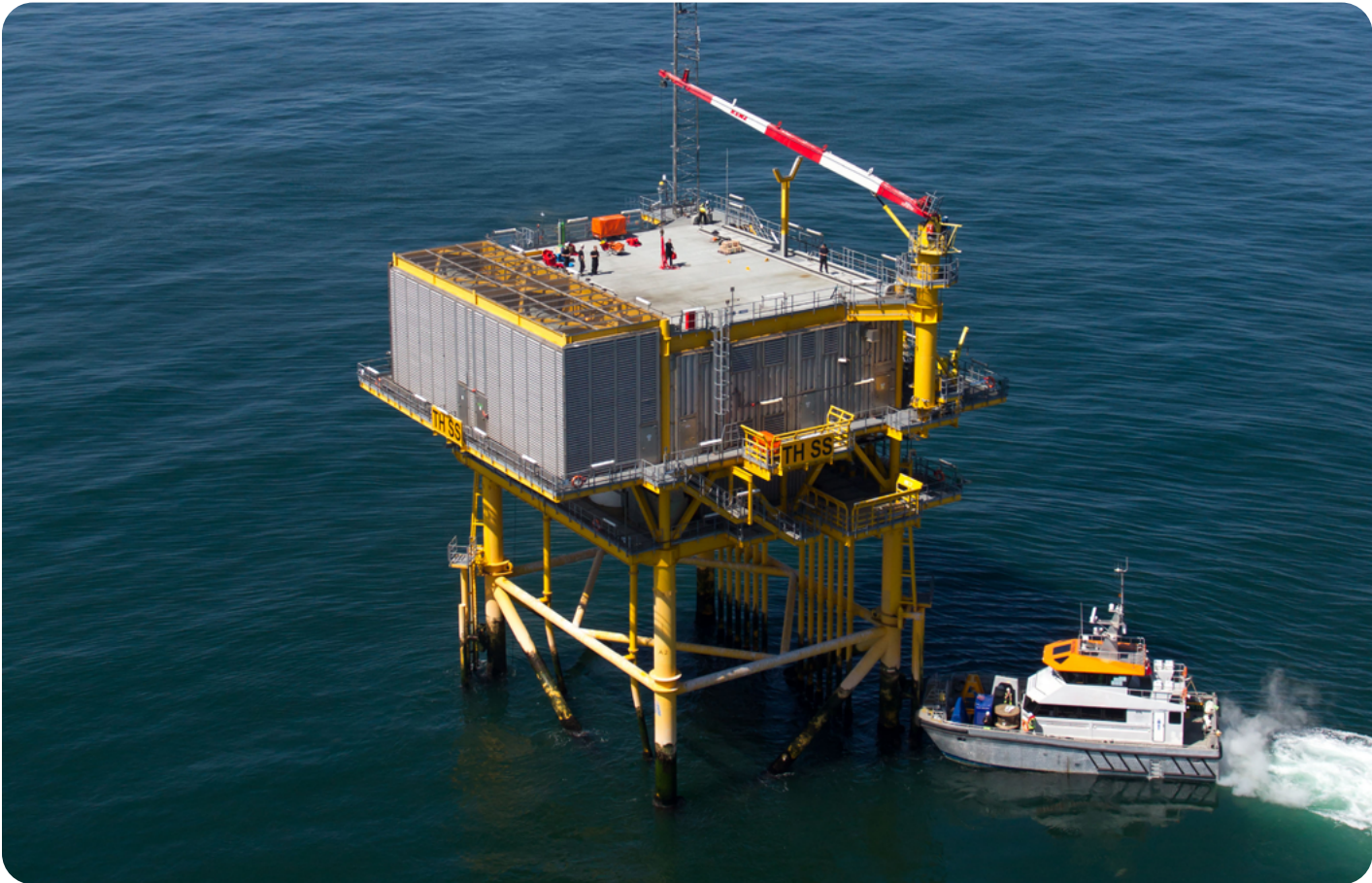
Offshore substations are critical connection points between the grid and offshore renewables.
