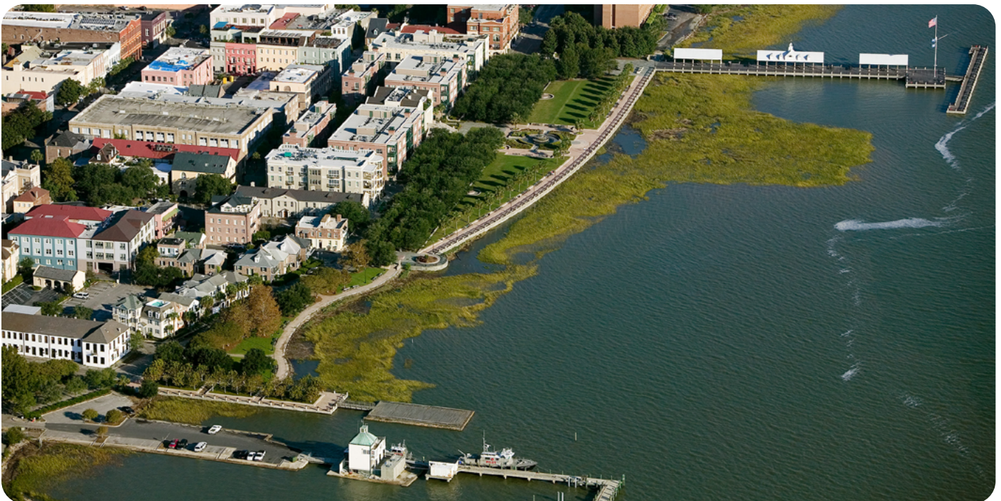
Charleston Waterfront Park project created new access points to the Cooper River in Charleston, South Carolina, restored salt marshes, and provided recreational opportunities for residents. Photo: Landslides, Courtesy of Sasaki
